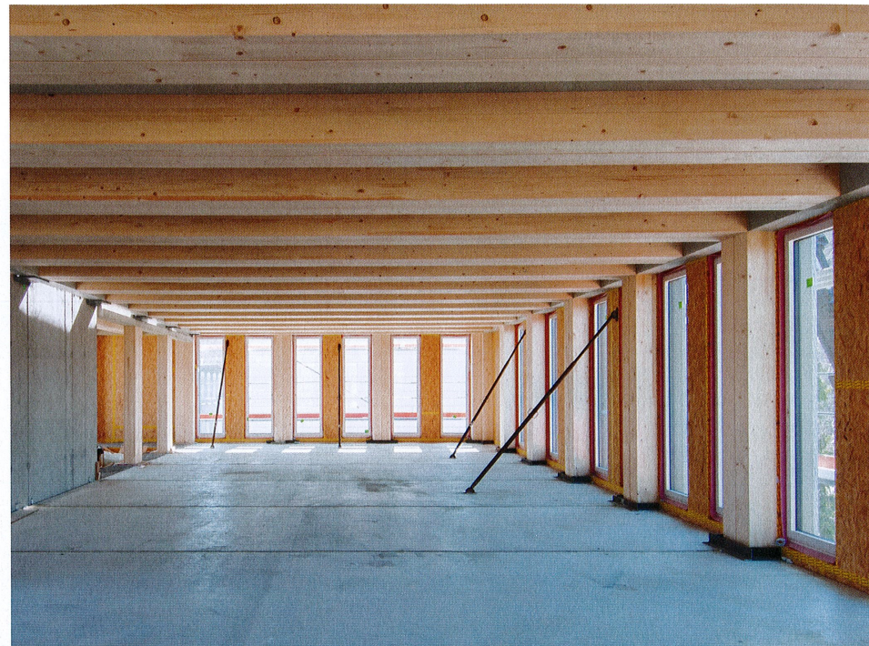
Above/left Life Cycle Tower One, Dornbirn, is designed by Hermann Kaufmann and engineered by Arup. The eight-storey building, constructed to Passivhaus standards, is the prototype for a high-rise timber construction system.
