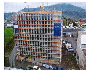
Above/left Life Cycle Tower One, Dornbirn, is designed by Hermann Kaufmann and engineered by Arup. The eight-storey building, constructed to Passivhaus standards, is the prototype for a high-rise timber construction system.
